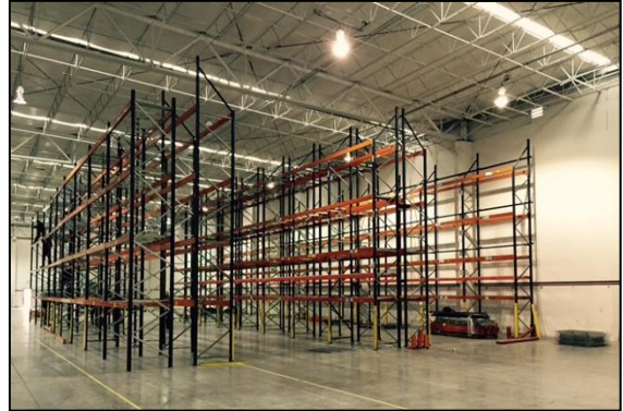
Distribution center under construction
